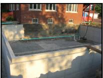
Work on the addition is in full swing as you can clearly see. Recap of work completed: Foundation wall poured, waterproofed and backfilled, perimeter drainage is in place,
